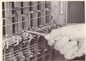
At the rear of the console remove the two retaining nuts which secure the component to be replaced.
